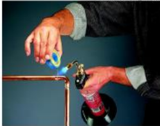
Afb. 17 Soldeerverbinding
